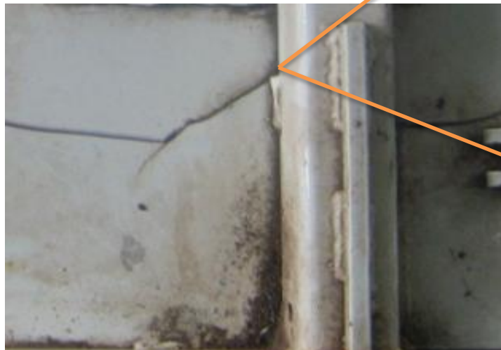
Vertical sheet cracked from weld toe
